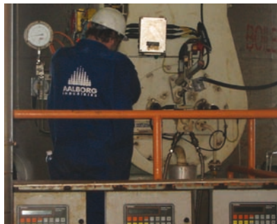
Service and upgrading of burners and safety/control systems
